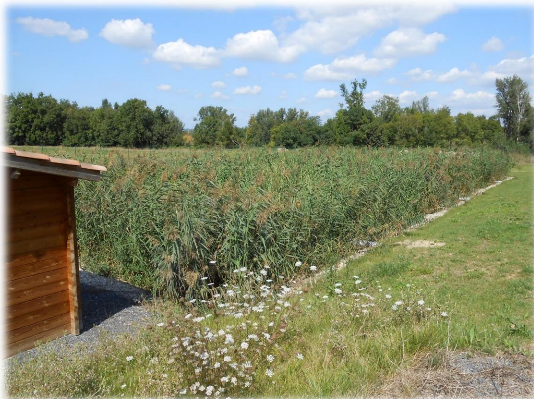
Figure 2. Aspect of a Vertical Flow Constructed Wetland located in Toulouse (France).
